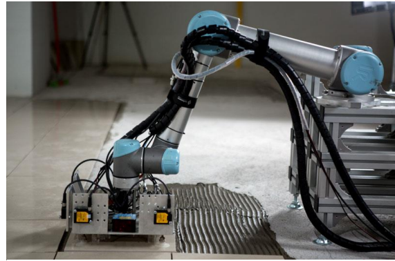
Figure 16: 3D laser imaging based robotic applications for laying floor tiles
